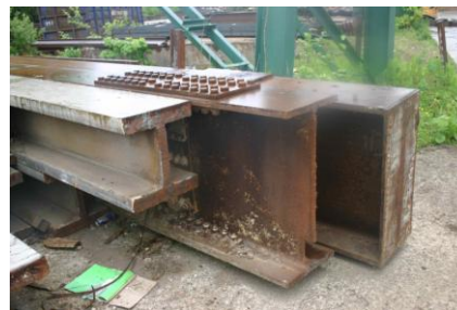
Figure 5: Reclaimed Structural I-Beams
